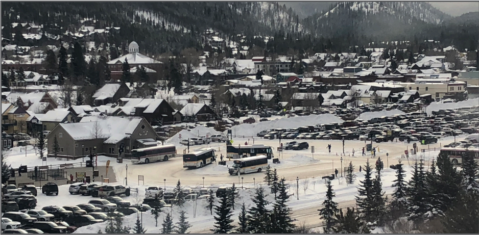
Breckenridge Station Transit Center for Free Ride, Summit Stage, resort, and hotel shuttles
